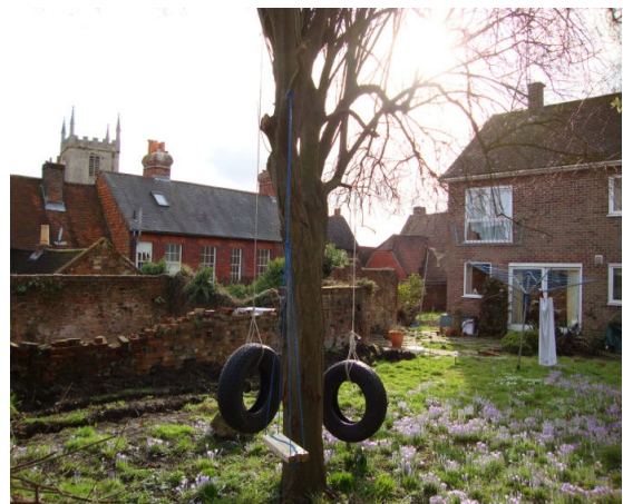
View of part of the rear elevation
